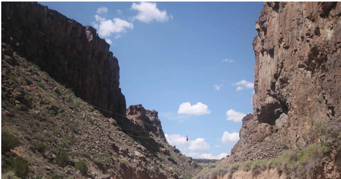
Figure 5 Track line geometry in lower Diablo Canyon. Span length = 84 m, slope = 11 degrees. Red dots are the location of the anchor.
