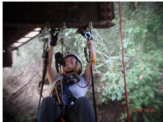
**Photo 12: Bridge Truss Floorbeam Inspection**
