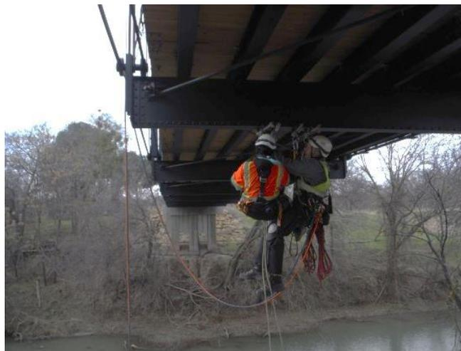
**Photo 13: Rescue from beam clamps in progress. Adjacent set of lines being used.**
